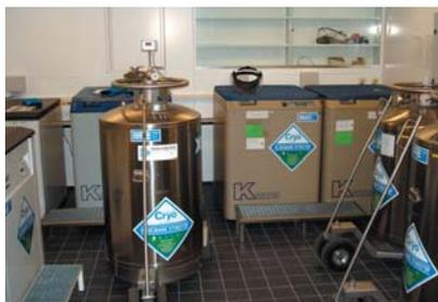
Having previously supplied Erasmus MC Hospital in Rotterdam with its cryobanks, Cluster 6 has now also opted to purchase a completely new cryobank from Cryo Solutions. The project comprises vacuum insulated piping and a PLC control unit which contains a switch over device and a de- gas and simultaneous filling system.
