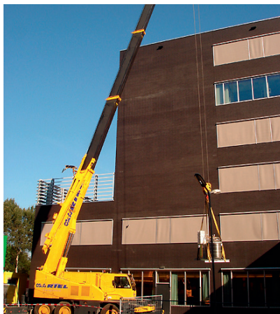
Pressure vessels are hoisted
